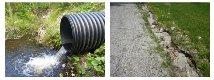
**Figure 4:** The AOP barrier created by a perched 48" culvert along South Road (left) was the lowest scoring projects (SC-2). The extreme erosion along the edges of Barney Orchard Road (right) was the highest scoring project (RD-8).
